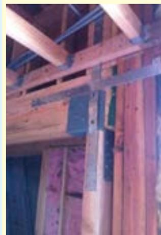
The typical sheet metal strapping that was required by the City though the building
