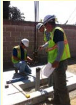
The electricians installing the new SCE transformer pad
