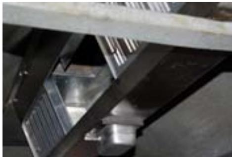
*The new stainless steel grease filter trays*
