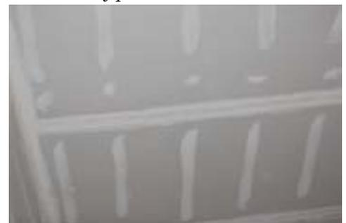
*Interior of the elevator shaft with gypsum board and taped*
