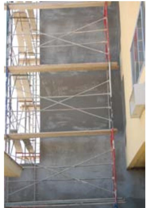
*The exterior of the elevator shaft with its scratch coat of plaster*
