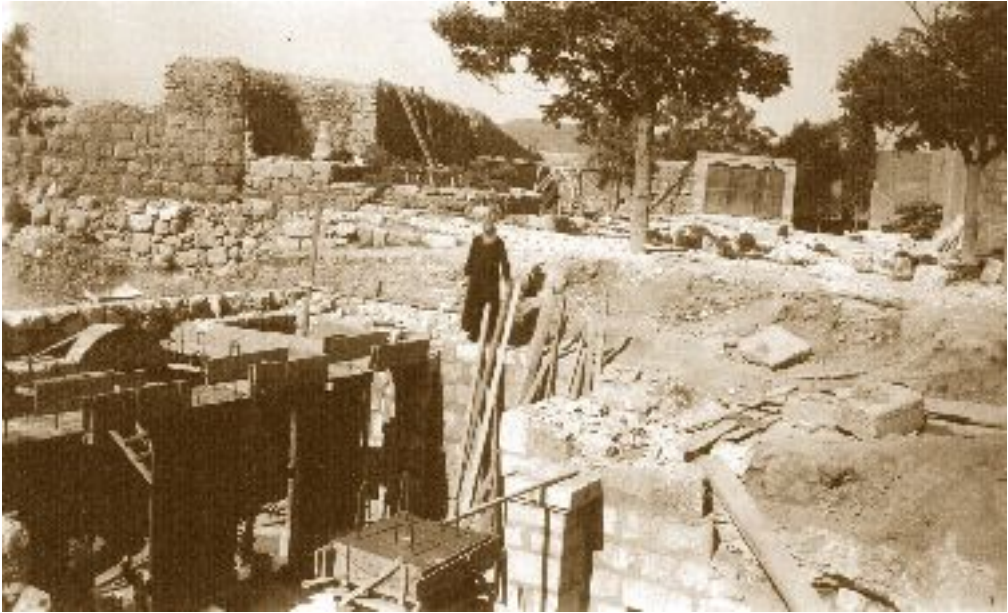
Autumn 1929: Fr Bianchi inspects building works at the Martyrium
