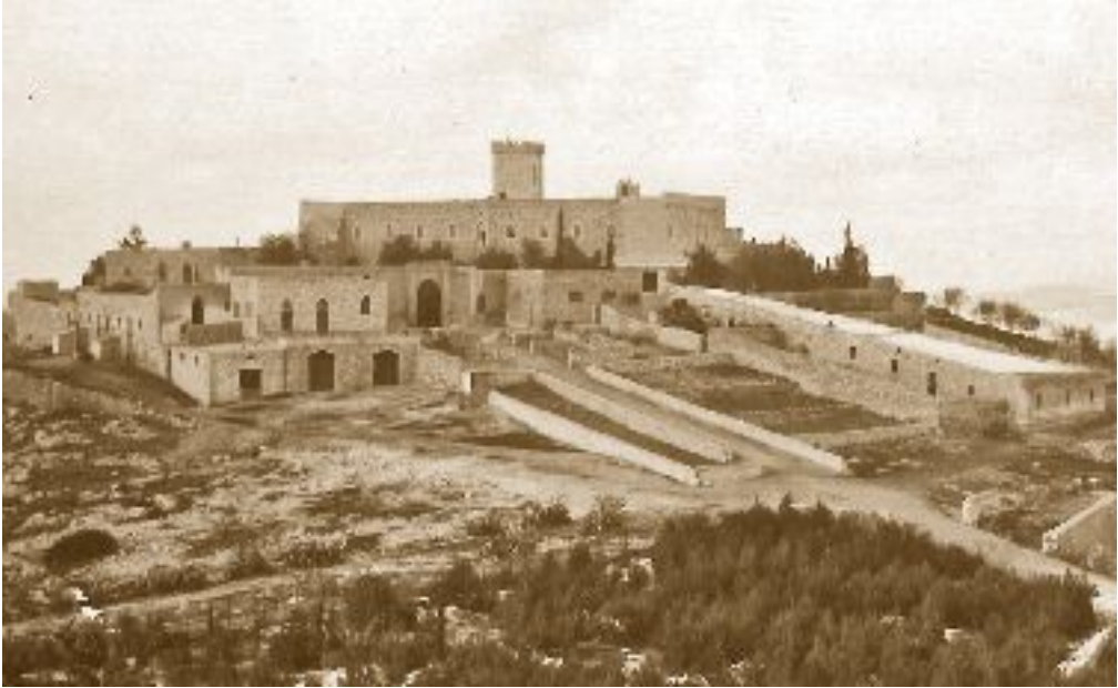
General view after 1931. East: peasant houses and barns. South-Est: driveway; on left: garages, stores, electricity hub. Above: terrazzo with balcony in front of the school and clinic. South: mill and press; N-W the FMA house.
