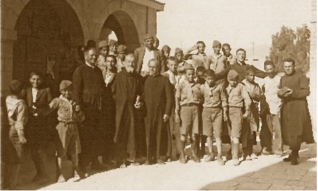
Final visit of Fr Maurizio Gisler osb, in front of the Martyrium for which he was architect (03.08.1939).
