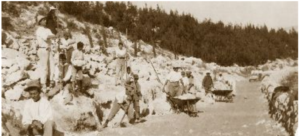
Early 1930s: excavation of the rocky ridge under the barn to widen the road.
