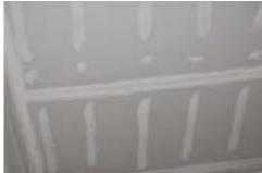
Interior of the elevator shaft with gypsum board and taped
