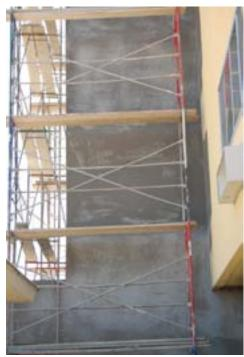
The exterior of the elevator shaft with its scratch coat of plaster
