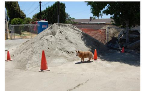
*Pile of sand: NB: the bottom of the electrical conduit trenches, there must be 6 inches of sand mixed with pee grave as a base for the conduit pipes another 6 inches on top of the pipes before the back fill takes place*
