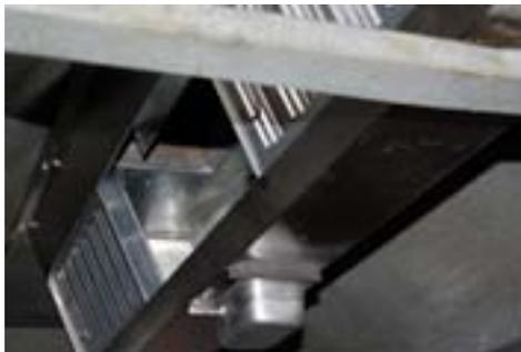
*The new stainless steel grease filter trays*
