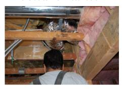
Wrapping the ventilation duct with installation
